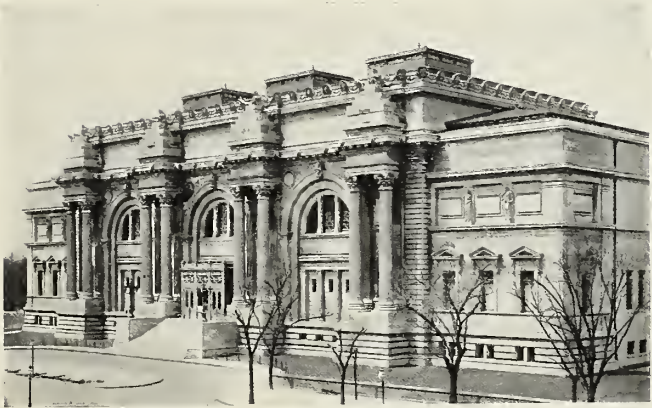
EAST WING OF THE MUSEUM AS COMPLETED
